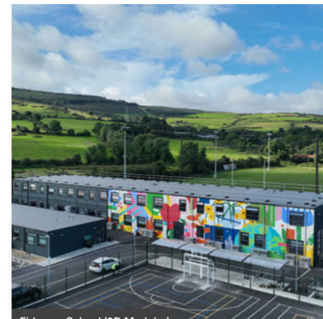
Firhouse School (3D Modular)
