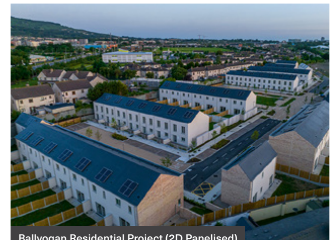
Ballyogan Residential Project (2D Panelised)
