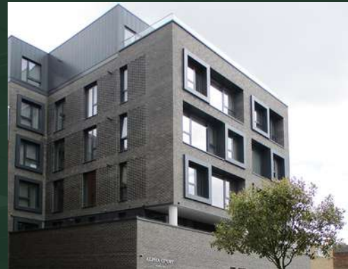
Station Road Housing £3.3 m
